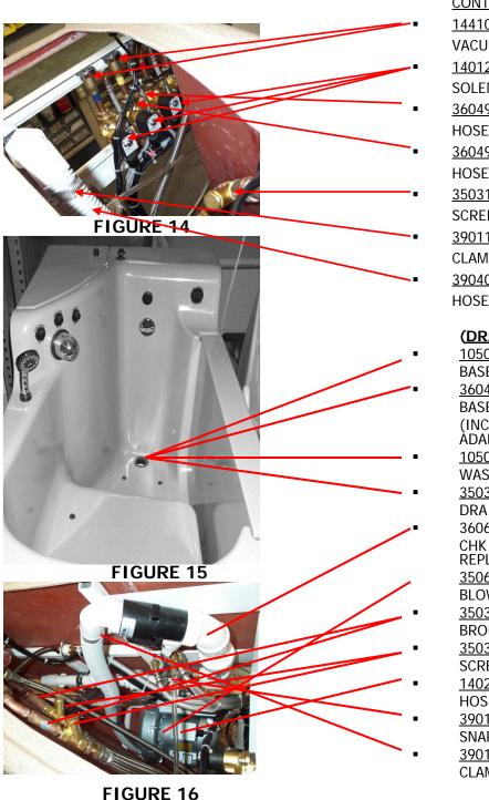
CONTINUED 144105 VACUUM BREAKER 140124 SOLENOID VALVE 360492 HOSE - 3/8" X 60" SS 360491 HOSE - 3/8" X 48" SS 350315 SCREEN MESH IN-LINE 390112 CLAMP HOSE SS 390409 HOSE VAC 1-1/4 ID (DRAIN PARTS) 1050401 BASE SHOE BASKET 360402 BASE SHOE ASSY (INCLUDES SHOE AND PLST ÀDAPT) 1050345 WASHER RUBBER 350391 DRAIN SCREEN 360628A CHK VALVE 1 1/2" BLK SER REPLA 350602 **BLOWER** 350320 BRONZE CHECK VALVE 350315 SCREEN MESH IN-LINE 140261 HOSE 1/4" CLEAR 390111 SNAP CLAMP SIZE 390112 CLAMP HOSE SS
